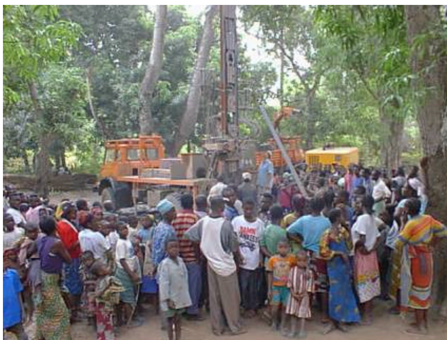
Figure 5.3 Community members standing too close to a drilling rig for safety.
