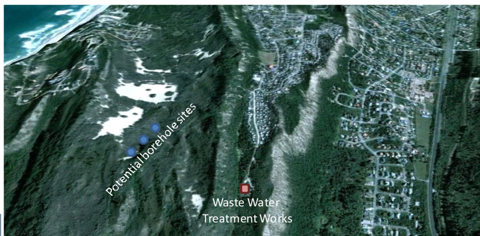
Aerial photograph of Sedgefield WWTW in the sand dunes and proposed abstraction boreholes (Google Earth, 2010)
