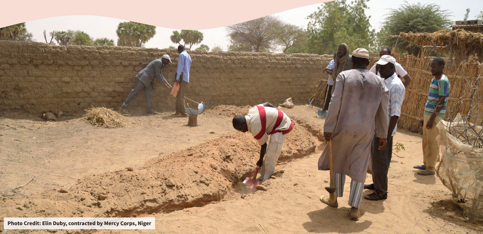
Digging an on-contour swale
