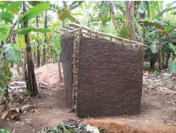
Sexual violence against women can be reduced drastically when gender sensitive decisions are made about location, privacy and other features of sanitation facilities.
